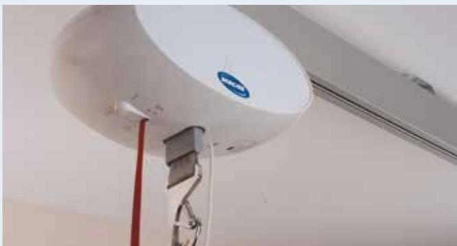
**Single track systems** take a patient to and from fixed points along a single straight, angled or curved track (this can also be mounted on a gantry A-frame system for temporary use).
